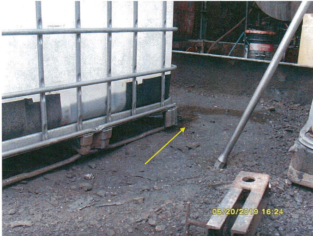
Photo 7 (SI851032): A tote of unknown petroleum chemical actively leaking onto the ground at the time of inspection (leaked fluid indicated with yellow arrow). The area smelled strongly of petroleum. Facility representatives placed clean absorbent pad under the leak after Mr. Dobrowski pointed it out to them.
