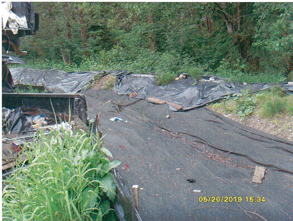
Photo 14 (SI851003): Western view of the trench and berm at the north end of the facility yard.
